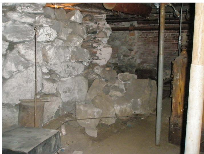
Before and After views show progress on repairs to the collapsed foundation wall.
