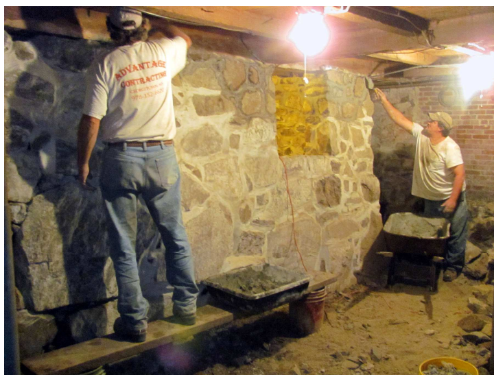
Before and After views show progress on repairs to the collapsed foundation wall.
