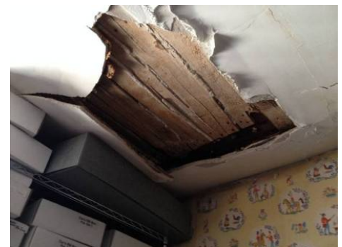
Collapsed section of ceiling at museum
